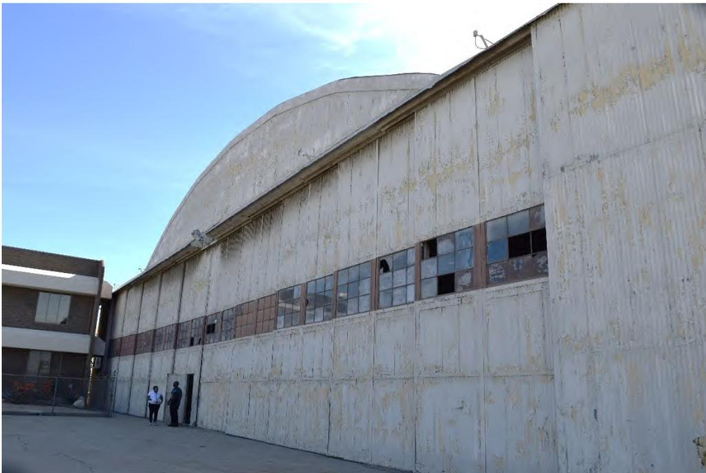
Building 3, northwest elevation. Note intact original siding, doors, and windows.
